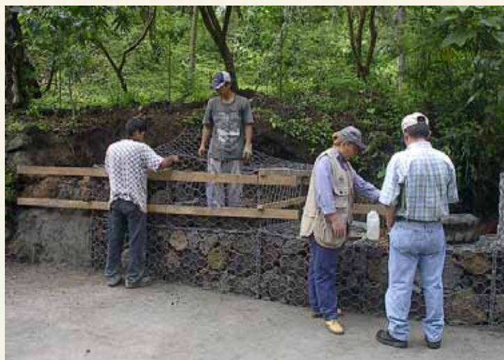
Roadside retention wall in Berlín
